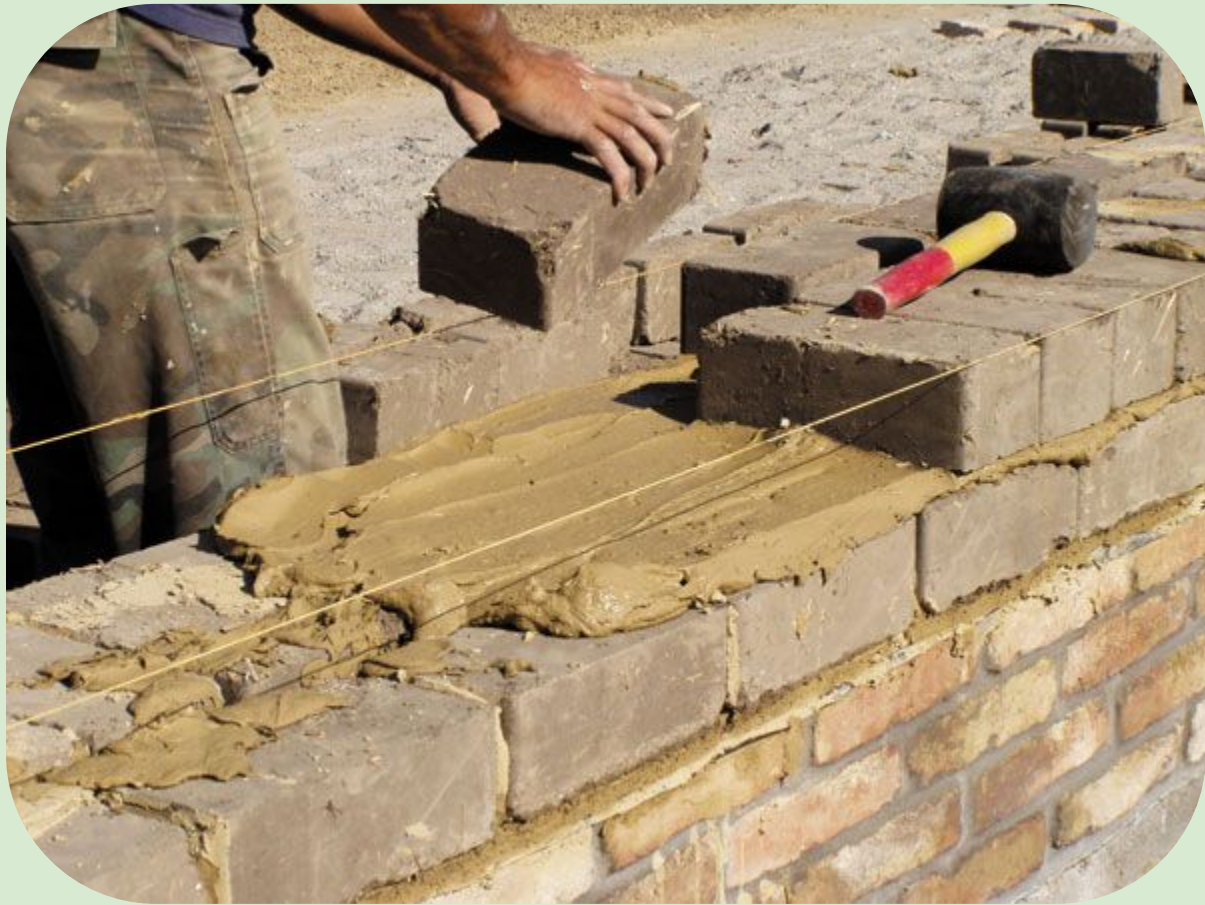
Building with mudbricks
